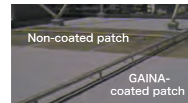
▲Comparison of GAINA-coated and non-coated patches on RC structure roof Test date: September 3, 2008 External temp: 33°C (91°F)
